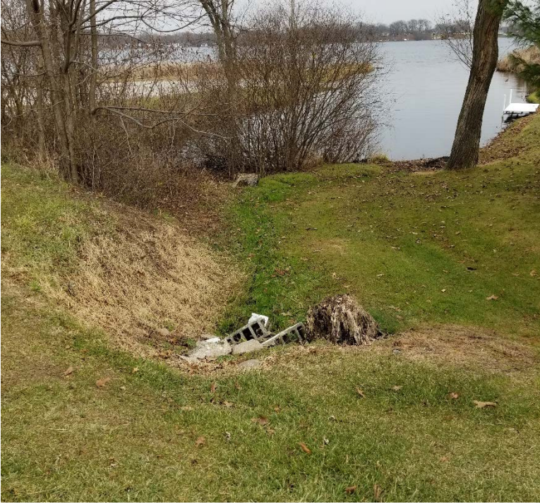
Figure 29. Photo of eroding catch basin spillway on east-side of CR 890 E, near the public access.
